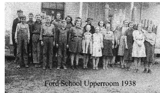
Ford School, 1925-1950, Schoolhouse Lane, Ford, Ky. portions of this school are behind a modern front.
