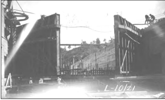
Lock gates at No. 10
