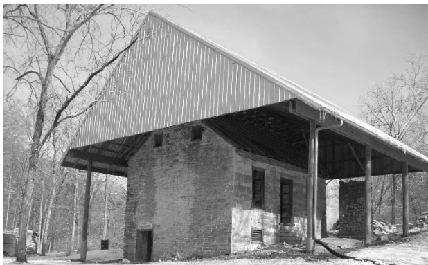
Jonathan Bush house in the Preserve
