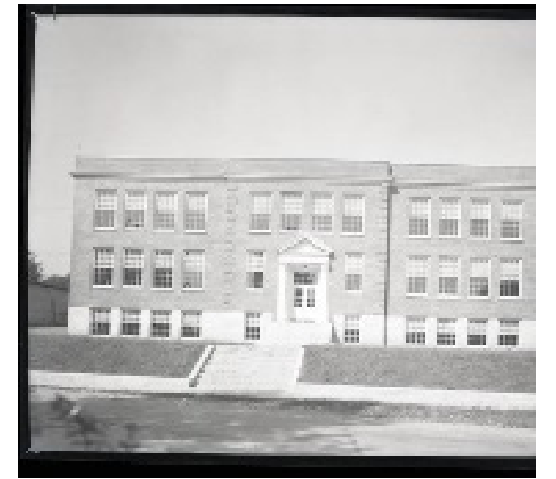
Oliver Street Colored School, 1940 (photo by Ogden), built by WPA in late 1930s.
