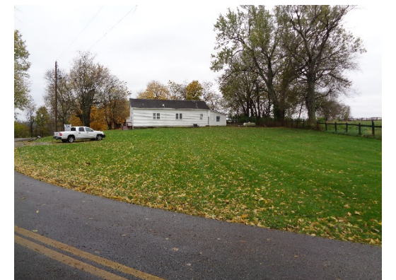
Becknerville Colored School, 1899-1930, 3150 Waterworks Rd.
