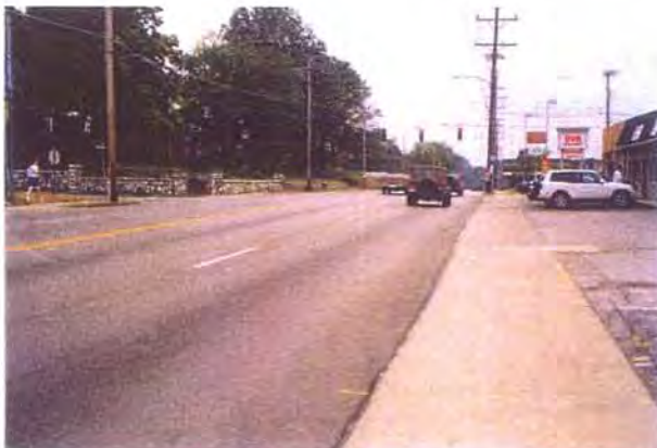
Figure VI- 5. Poor Roadway Edge Delineation
