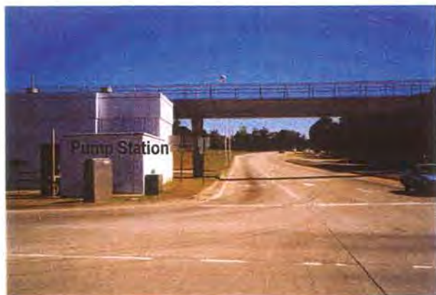
Figure VI- 3. Wilkinson Boulevard Pump Station
